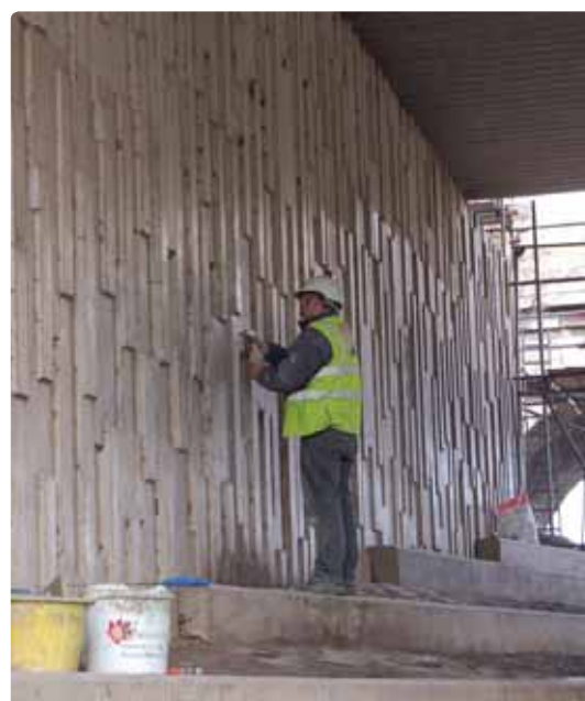
Figures 7 and 8 left: Concrete repair operations to figured abutments.
