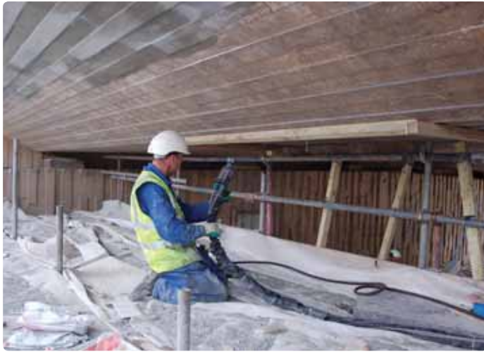
Figures 1 and 2 above: Concrete repair operations to soffit of bridge.
