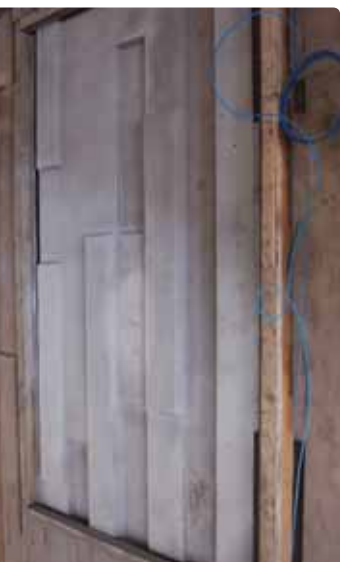
Figure 3: Trial CP area using thermal arc spray material.
