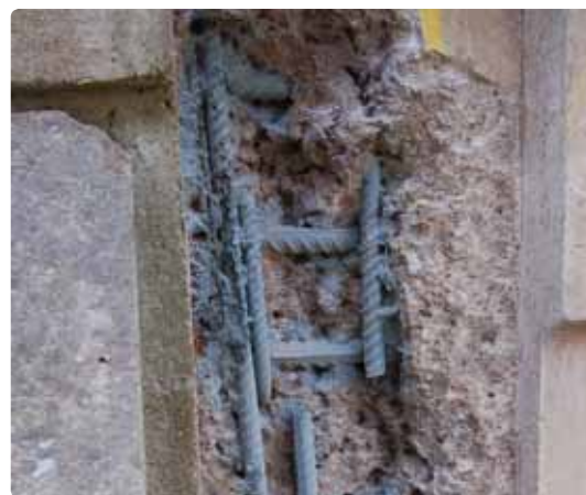
Figure 6 left: Prepared steel within repair area to abutment.
