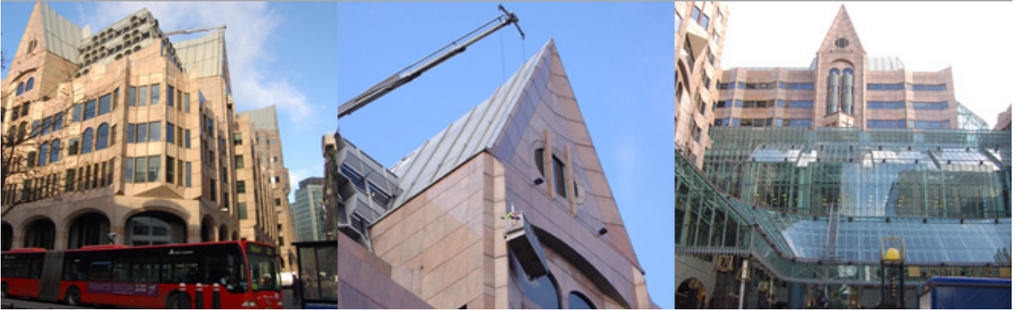
Cleaning to External Granite Facade using Cradles
