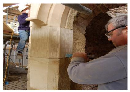
Stone restoration repair options are broadly the same as those used for other types of masonry and include complete renewal, insitu surface restoration, or consolidation.
